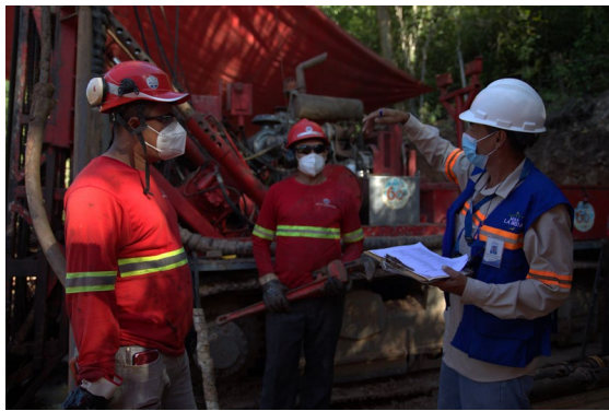
Diamond core drilling rig inspection with contractors Rodio-Swissboring.
