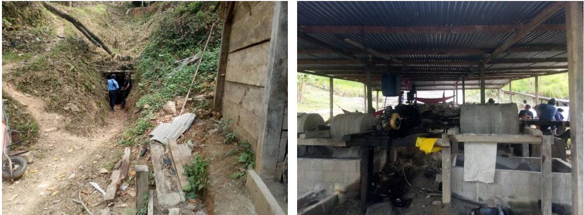
Figure 14. An adit driven into the base of the ridge to exploit the Northwest structure (left). Ball mills processing the ore.
