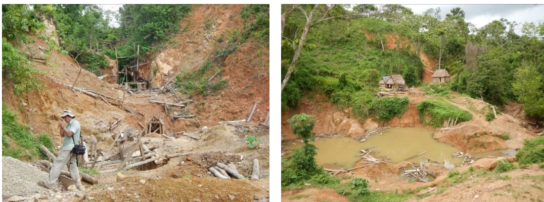
Figure 13. Collapsed and flooded artisanal mine workings following the first rains of the wet season in May. Photograph taken from the same location looking southwest (left) and northeast (right) along the strike of the mineralisation.
