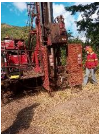
Start of drilling LIWB584
