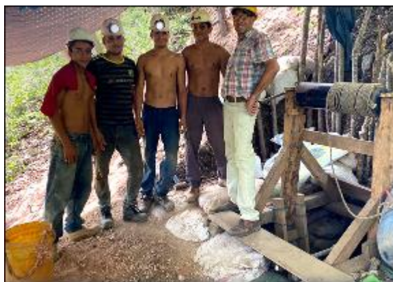
Inspection of work in the Espinito Mendoza area.
